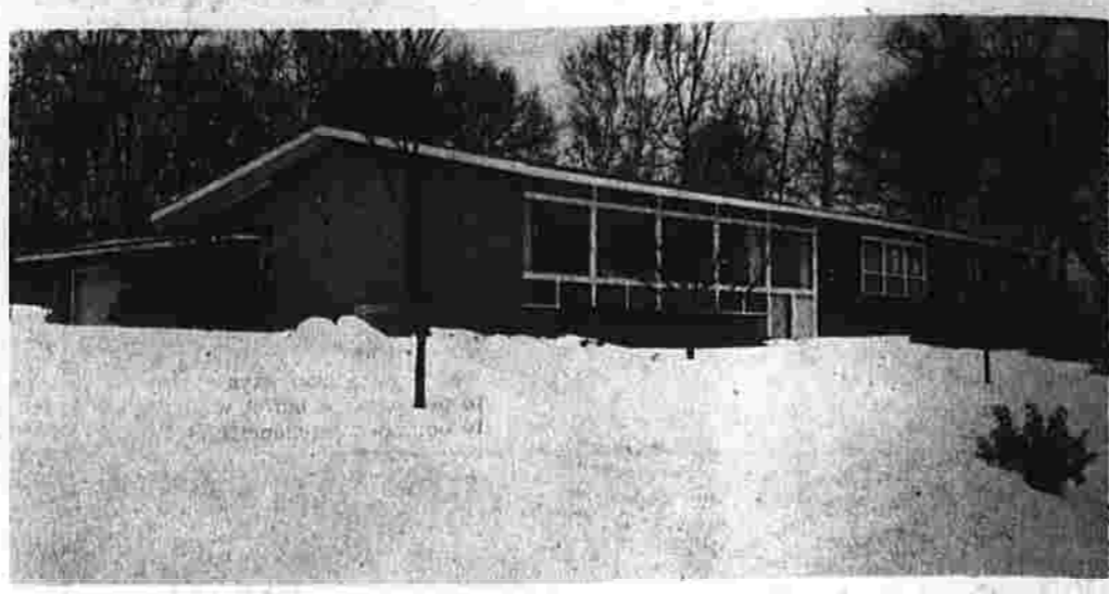
The Walter Ferguson hilltop residence at 104 Garth Rd.
